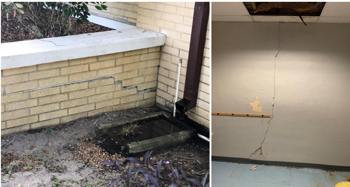
Structural damage visible from the exterior and interior of the Library building
